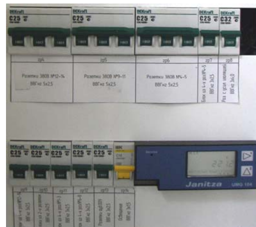
Fig 2. UMG 104 power analyzer (data collector) installed into lighting control panel
